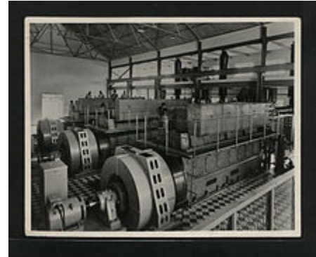
Three English Electric 7SRL diesel-alternator sets being installed at the Saateni Power Station, Zanzibar 1955
