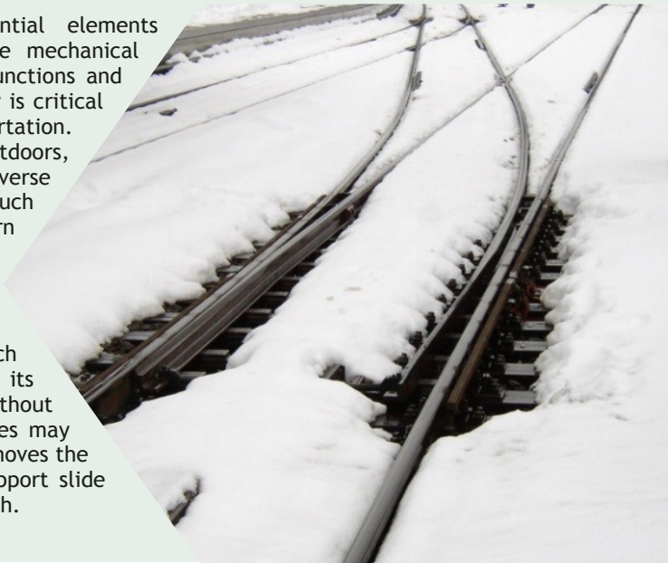
Figure 1: Railway switch with gas heater. Source: Fabian Grunder. Wikipedia Commons.
