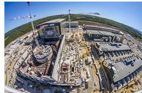
ITER, currently under construction, will be the largest tokamak by far.
