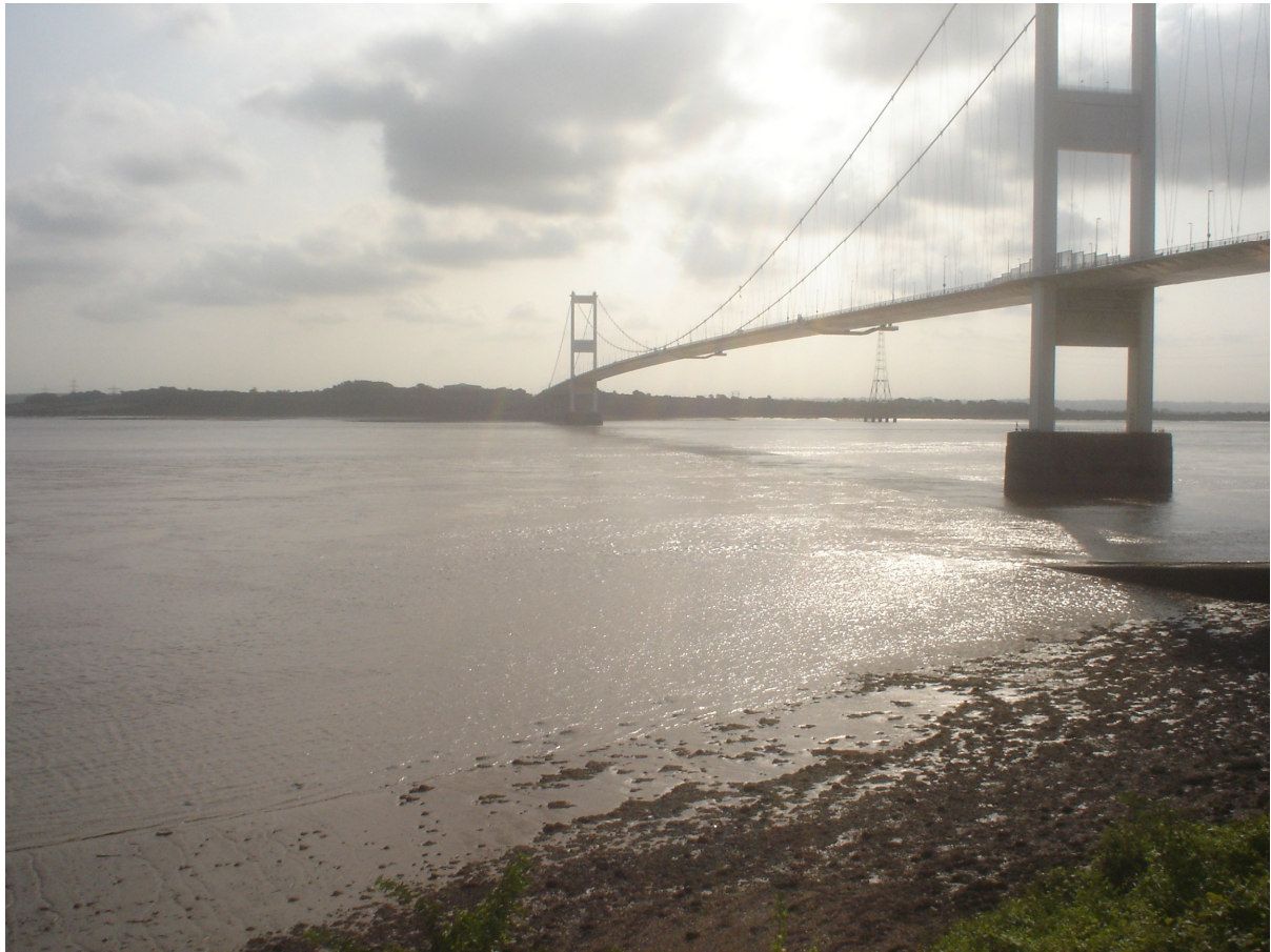
Figure 12: Second Severn crossing – near the site of the proposed Beachley barrage
