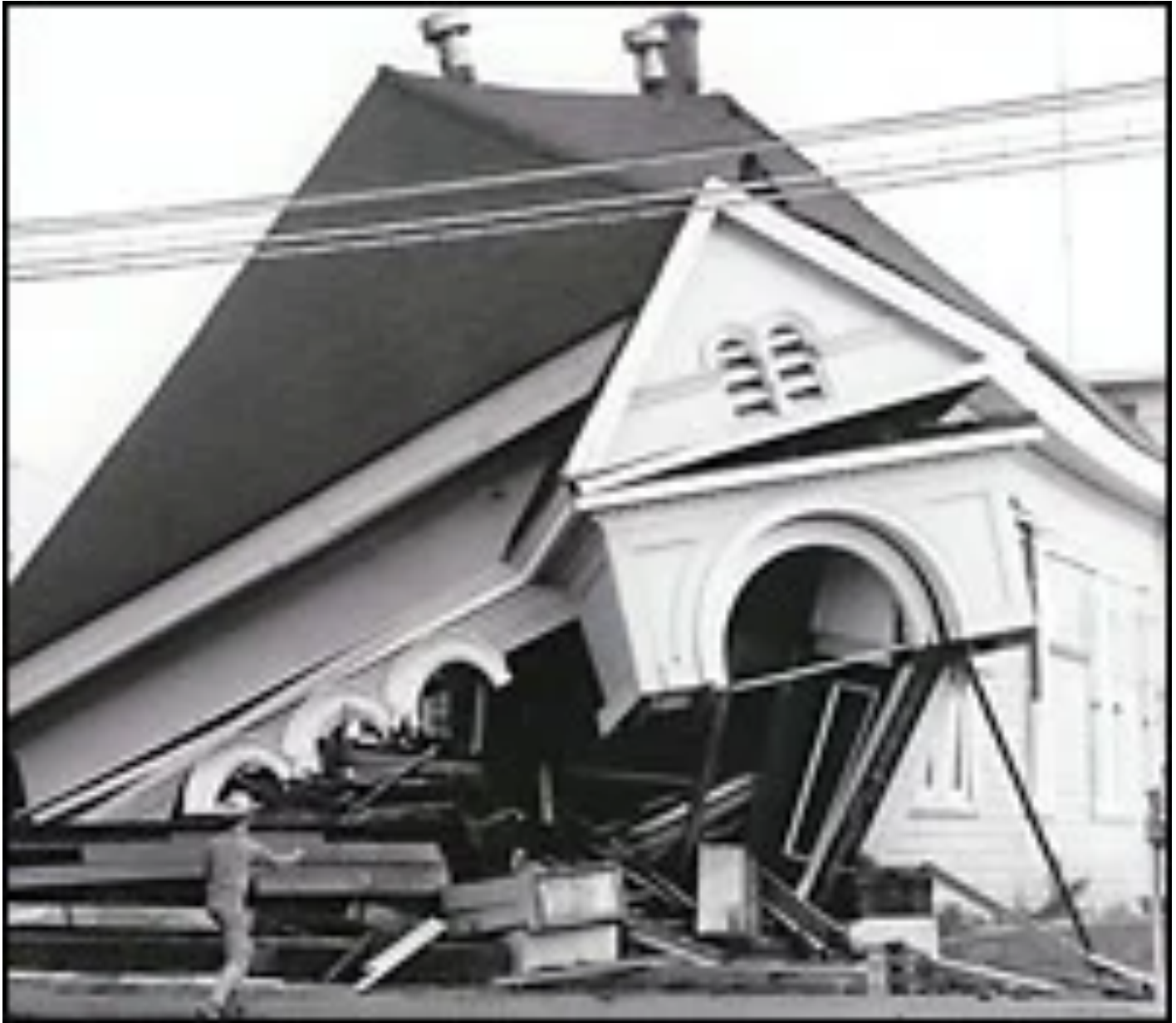
A damaged law office.
