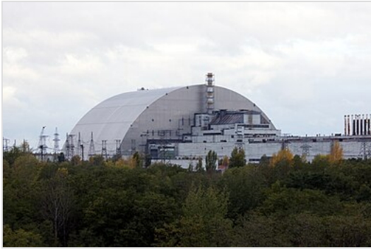
New Safe Confinement in 2017.
