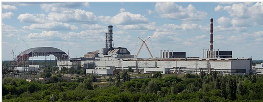
A stitched panorama view of the Chernobyl Nuclear Power Plant site in Ukraine, pictures taken in June 2013. Descriptions of the buildings from left to right: First half of the New Safe Confinement (under construction) after second lifting operation (had not yet reached its final height), reactor 4 with existing shelter building and the new and old ventilation shafts, reactor 3, cranes to dismantle the old ventilation shaft, reactor 2, reactor 1.
