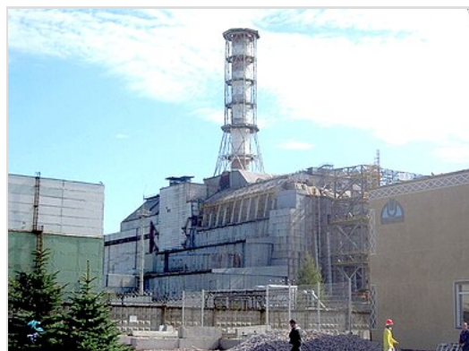
No. 4 reactor site in 2006 showing the sarcophagus containment structure ; Reactor No. 3 is to the left of the smoke stack
