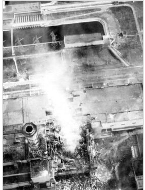
Steam plumes continued to be generated days after the initial explosion [39]
