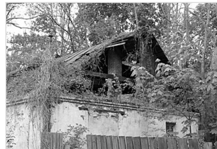
Ruins of abandoned house in Chernobyl (May 2019)
