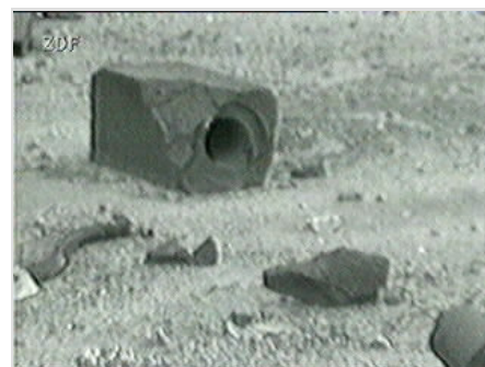
Video still image showing a graphite moderator block ejected from the core
