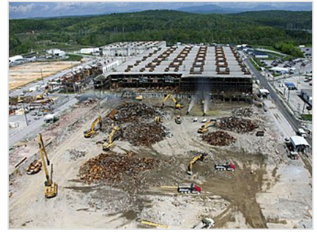
Demolition of K-25 in progress in April 2012
