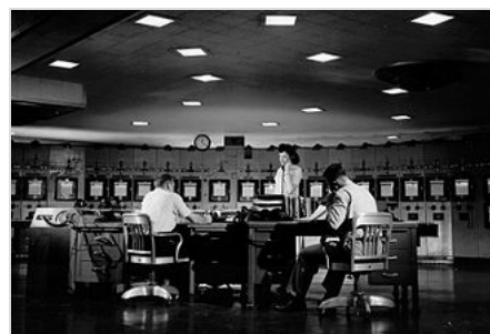
The K-25 control room
