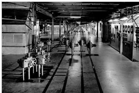
A worker on a bicycle in the K-25 operating level
