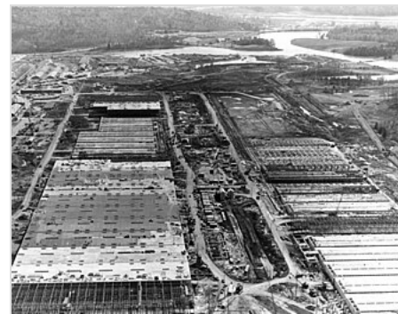
K-25 under construction
