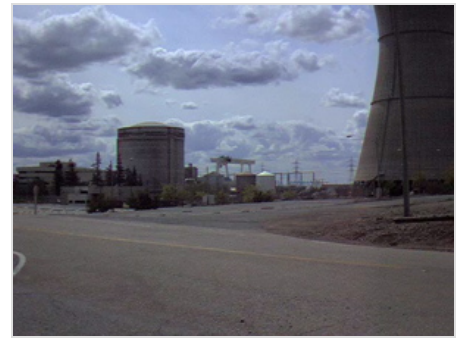
Rancho Seco PWR reactor hall and cooling tower (being decommissioned, 2004)
