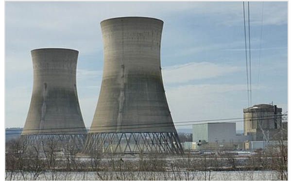
TMI-2 in February 2014. The cooling towers are on the left. The spent fuel pool with containment building of the reactor is on the right.
