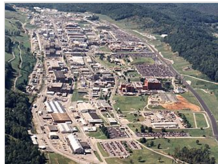
Y-12 National Security Complex in Oak Ridge, Tennessee.
