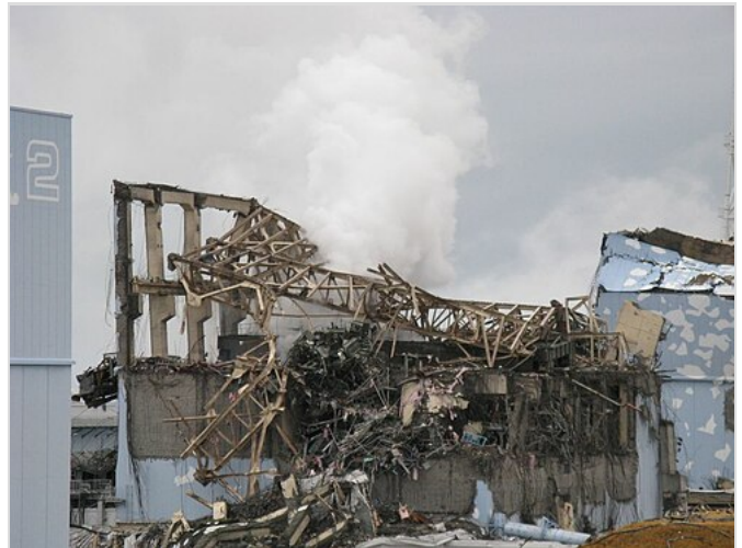
Unit 3 after the explosion on 15 March 2011 [55]
