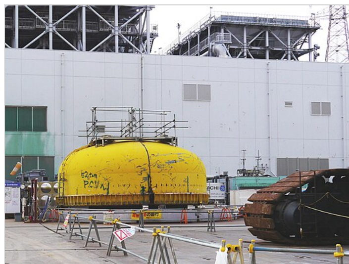
Top of Primary Containment Vessel, Unit 4 [56]
