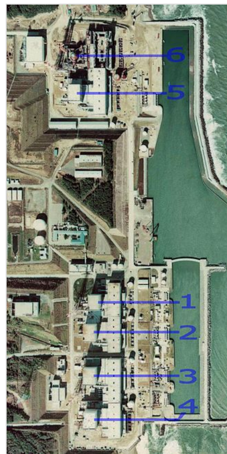
Aerial view of the station in 1975, showing separation between units 5 and 6, and 1–4. Unit 6, completed in 1979, is seen under construction. [24]
