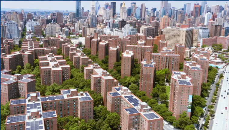
Where Tandem PV might supercharge this NYC complex: https://www.stuytown.com/sustainability/solar
