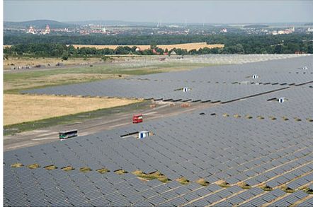
The utility-scale Waldpolenz Solar Park in Germany uses CdTe PV modules
