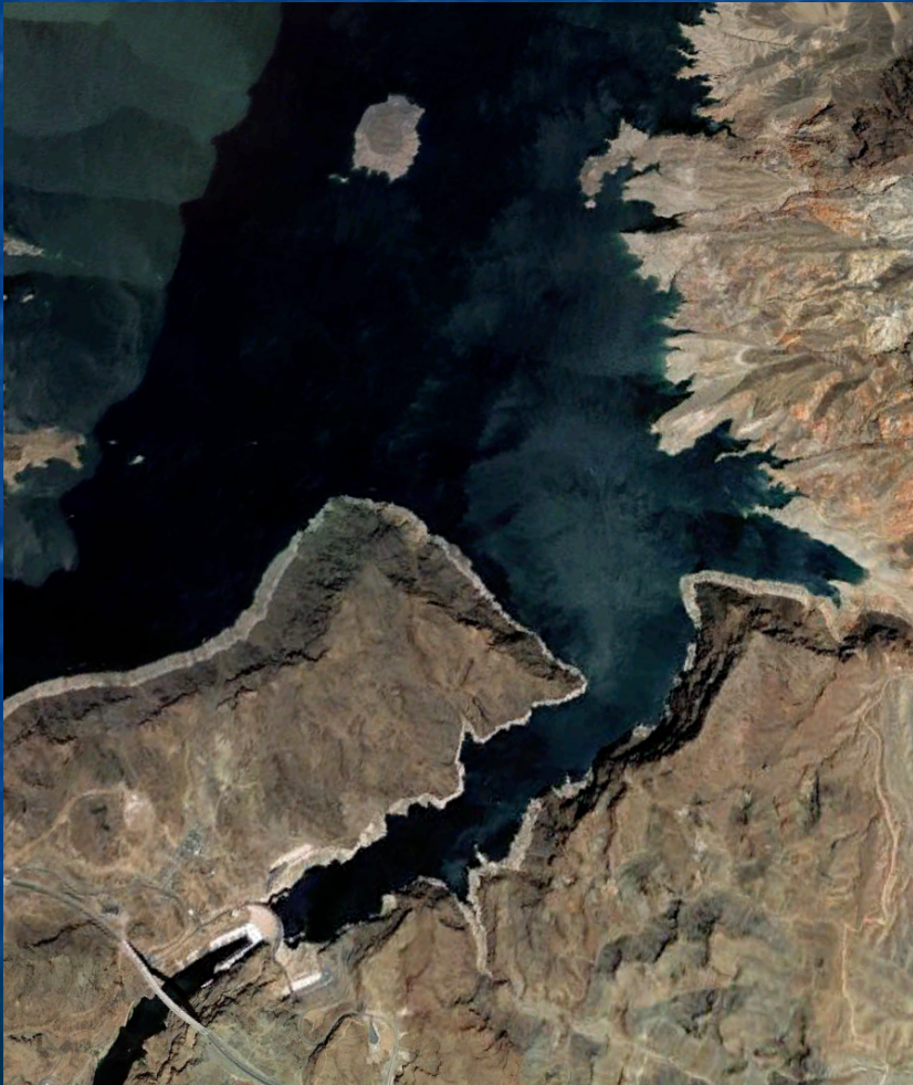
Hydro with Reservoir (Hoover Dam)
