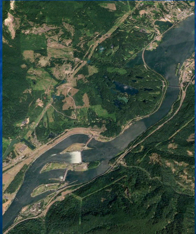
Run-of-the-River Hydro (Bonneville Dam)
