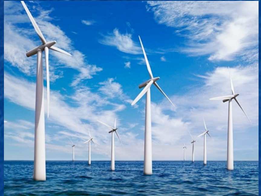
Offshore Wind Farm
