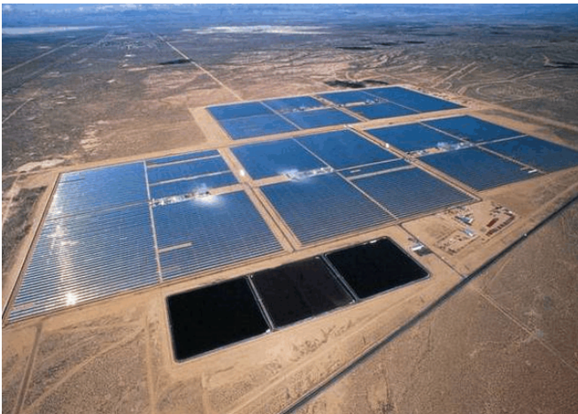
Figure 26. Representative Solar Thermal Plant: Nevada Solar One
