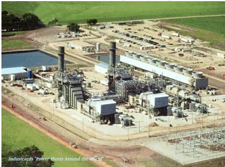
Figure 16. Representative Combined Cycle: McClain Plant (Oklahoma)
