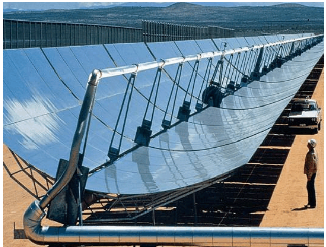
Figure 27. Nevada Solar One: Parabolic Collector Detail
