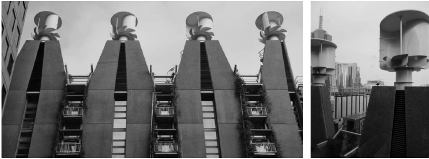
Figure 4: Savonius turbines used to assist ventilation and generate electricity on the Council House 2 (CH2) landmark building in Melbourne, Australia (photographs – copyright Pauline Anastasiou).
