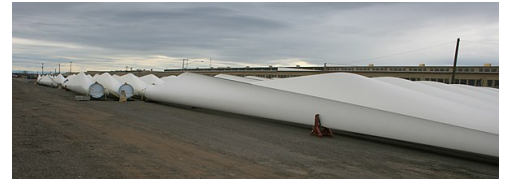
Wind-turbine blades awaiting installation in laydown yard.
